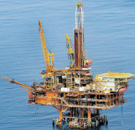
A state-of-the-art rig mounted platform RS-12 for expeditious production
