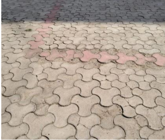
Paving Stone Installed in Campus
