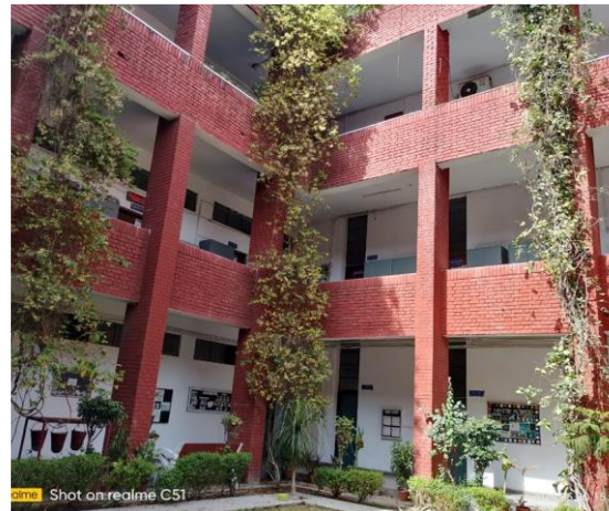
Well Ventilated Building
