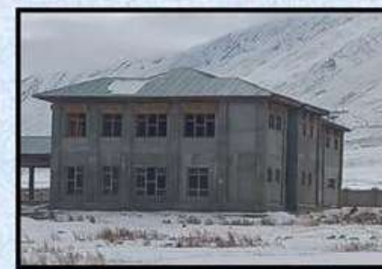
Administrative Block Work in Progress.
